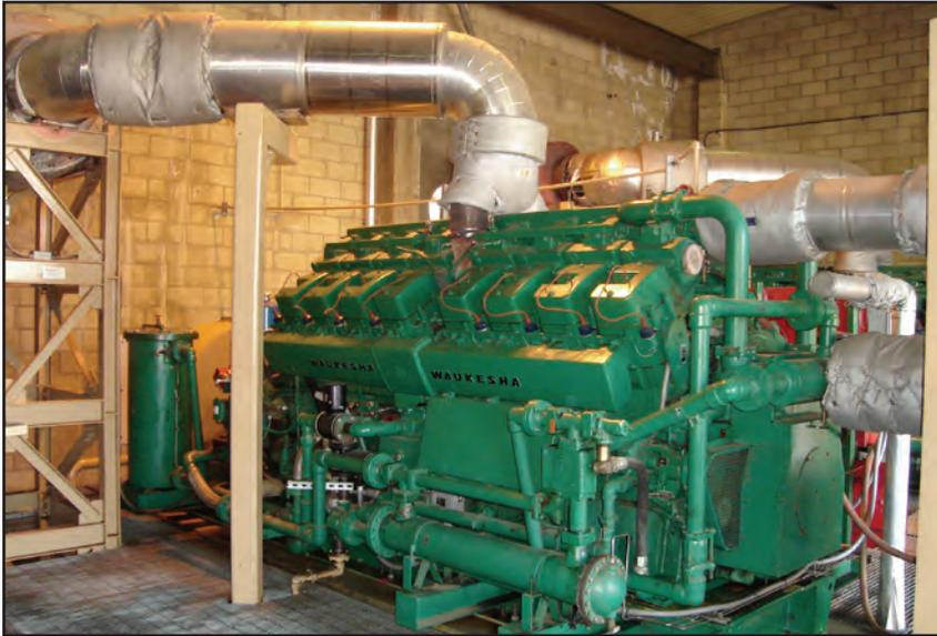
The County Sanitation Districts of Los Angeles County water treatment plant in Metro Los Angeles have installed Continental Controls Corp. ECV5 air/fuel control valves on five gaseous-fueled engines in an effluent pump station. The five new Waukesha Engine, Vee-configuration, 16-cylinder 9390 VHP units are each rated 1119 kW at 1200 r/min.
