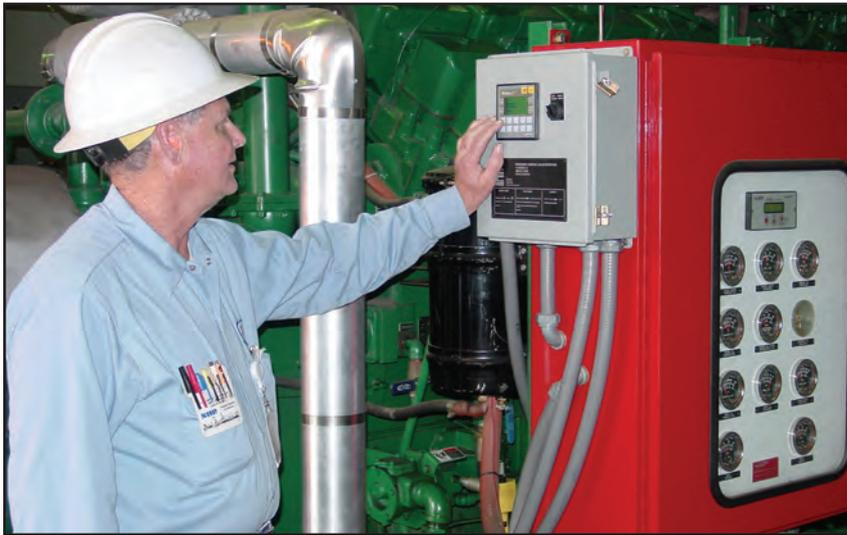
As part of the fuel system upgrade, 20 Continental Controls Corporation ECV5 air/fuel ratio control valves were installed on the five engines. Here, an engine technician checks O<sub>2</sub> set points on one of the engines via the ECVI display. To the right is one of the Murphy panels that allows technicians to monitor myriad temperatures and pressures for each engine.
