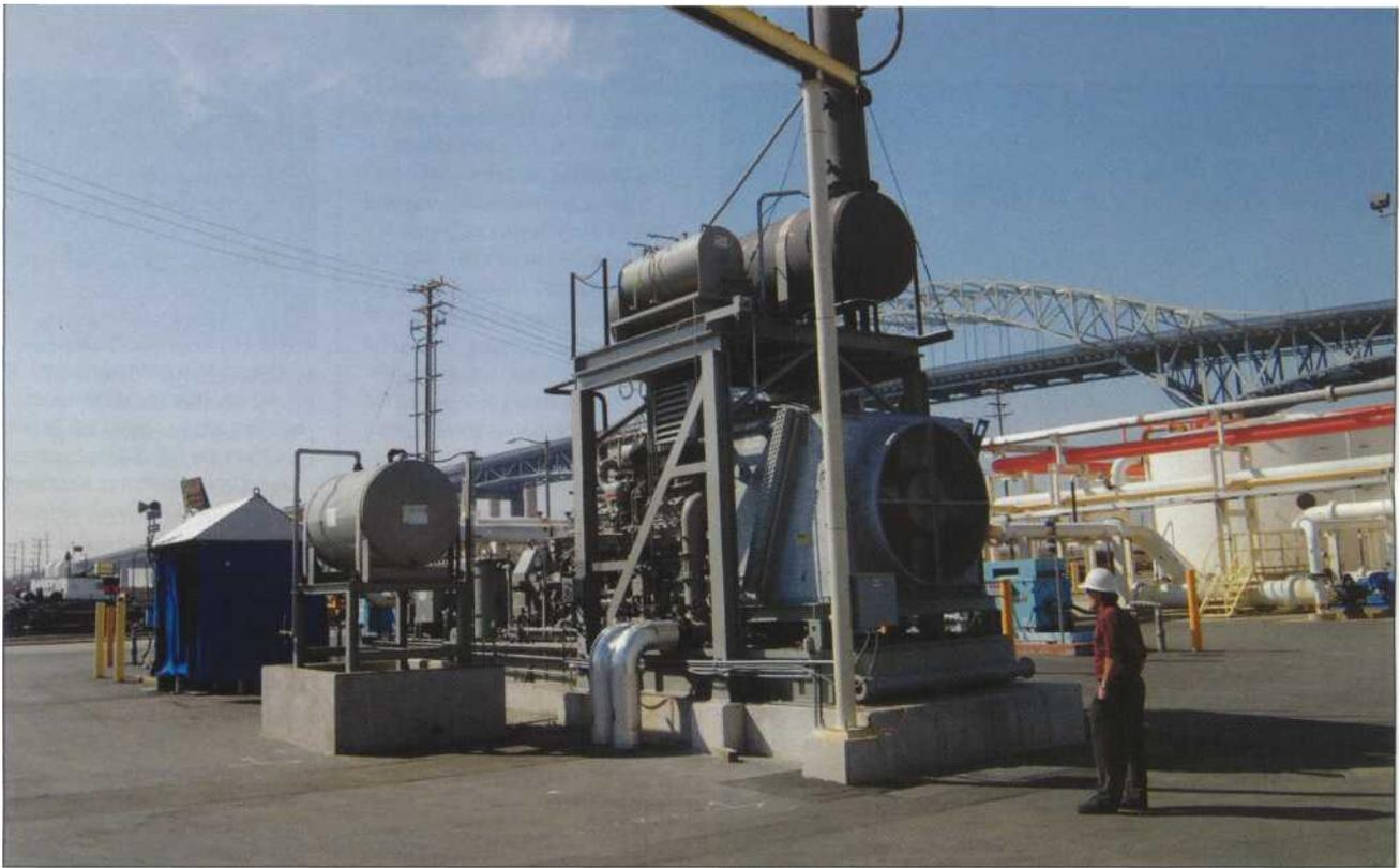
■ Tidelands Oil Production Company installed a Waukesha VHP P9390 GSI engine and pump package. The 2000 hp (1491 kW) natural gas-fueled engine drives a high-pressure centrifugal pump that's being used to inject water into several old oil reservoirs. The package replaced one of three electric motor-driven units previously used.
