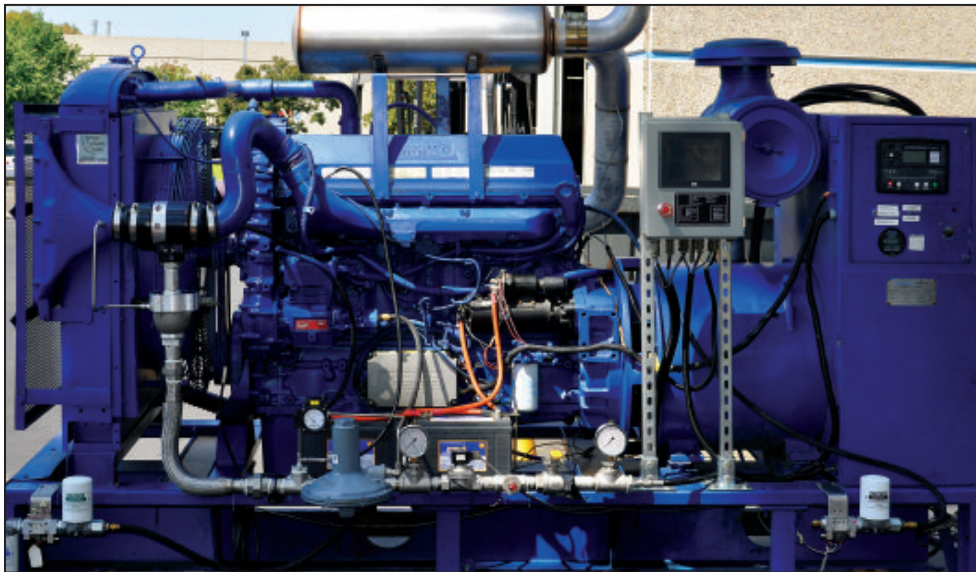
A Continental Controls GSS installed on a Detroit Diesel 60 series.
