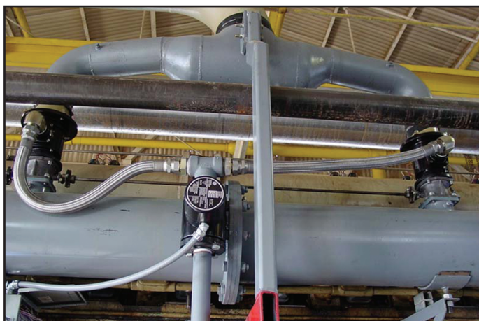
Continental Control Corporation converted the fuel control systems on two Enterprise GSG-8 engines at the Coalinga, California, U.S.A., crude oil pipeline station owned by ConocoPhillips Pipeline Co.
