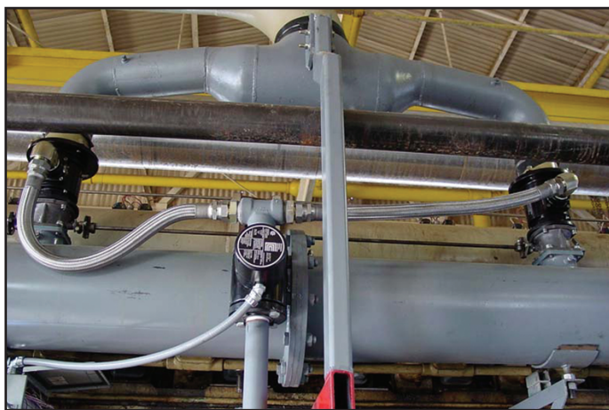
Continental Control Corporation converted the fuel control systems on two Enterprise GSG-8 engines at the Coalinga, California, U.S.A., crude oil pipeline station owned by ConocoPhillips Pipeline Co.
