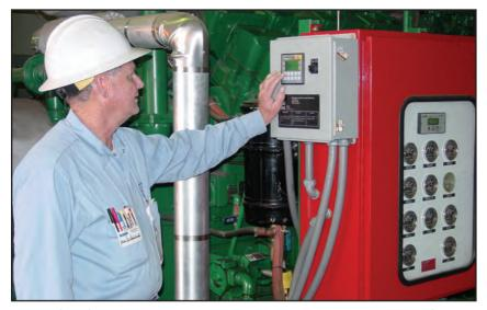
As part of the fuel system upgrade, 20 Continental Controls Corporation ECV5 air/fuel ratio control valves were installed on the five engines. Here, an engine technician checks  $O_2$  set points on one of the engines via the ECVI display. To the right is one of the Murphy panels that allows technicians to monitor myriad temperatures and pressures for each engine.
