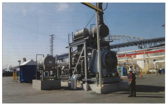
Tidelands Oil Production Company installed a Waukesha VHP P9390 GSI engine and pump package. The 2000 hp (1491 kW) natural gas-fueled engine drives a high-pressure centrifugal pump that's being used to inject water into several old oil reservoirs. The package replaced one of three electric motor-driven units previously used.
