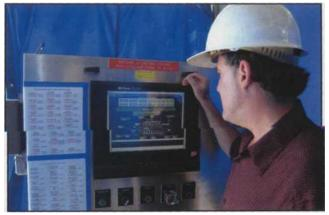
The entire engine and pump package uses a GE/Fanuc control system for overall control and monitoring functions.
