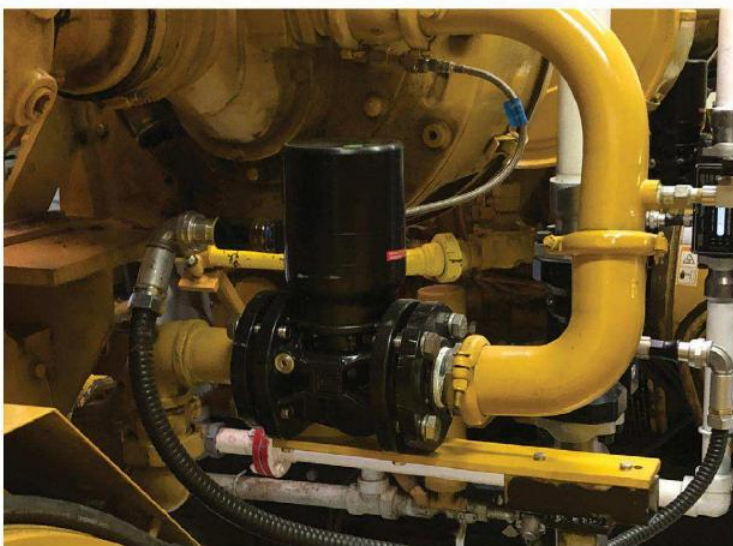
ECV 5 control valves along with a CCC FM 50 for measuring gas flow. Vortex routinely adds a FM 50 to check fuel consumption prior to adding the complete VETS system, then it provides fuel consumption after the upgrades. They report fuel savings of as much as 20% along with reduced emissions through the integration of the entire VETS system.
