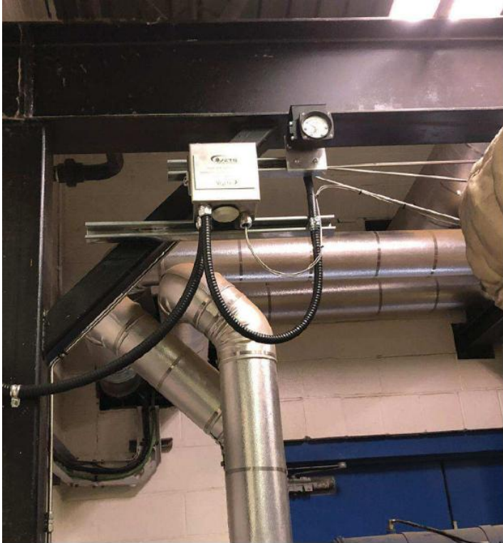
A Section Of The FM 50 Gas Meter Flow Measurement Device
