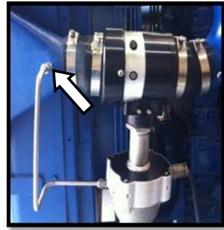
Figure 10 \frac{3}{8} " tubing for pressure reference.
